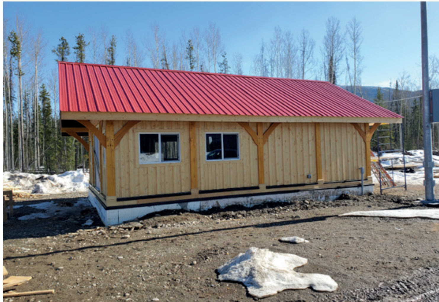
New waiting room at Fort Ware airstrip Photo Credit: Danny Case
